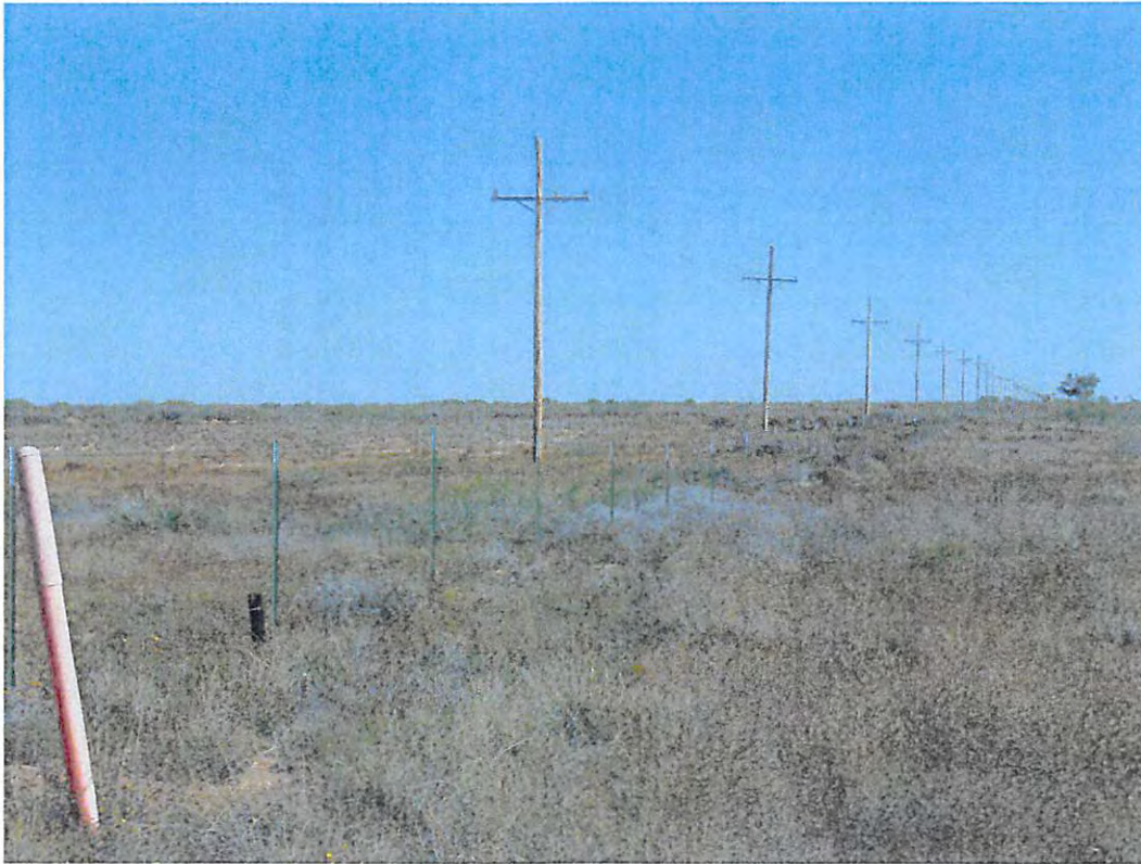
Power Lines Alongside and North of Clovis Highway
