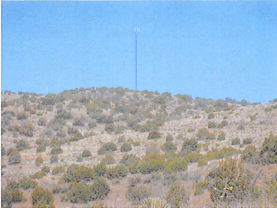
Closest Cellular Tower, 3.76 Miles to the Northwest
