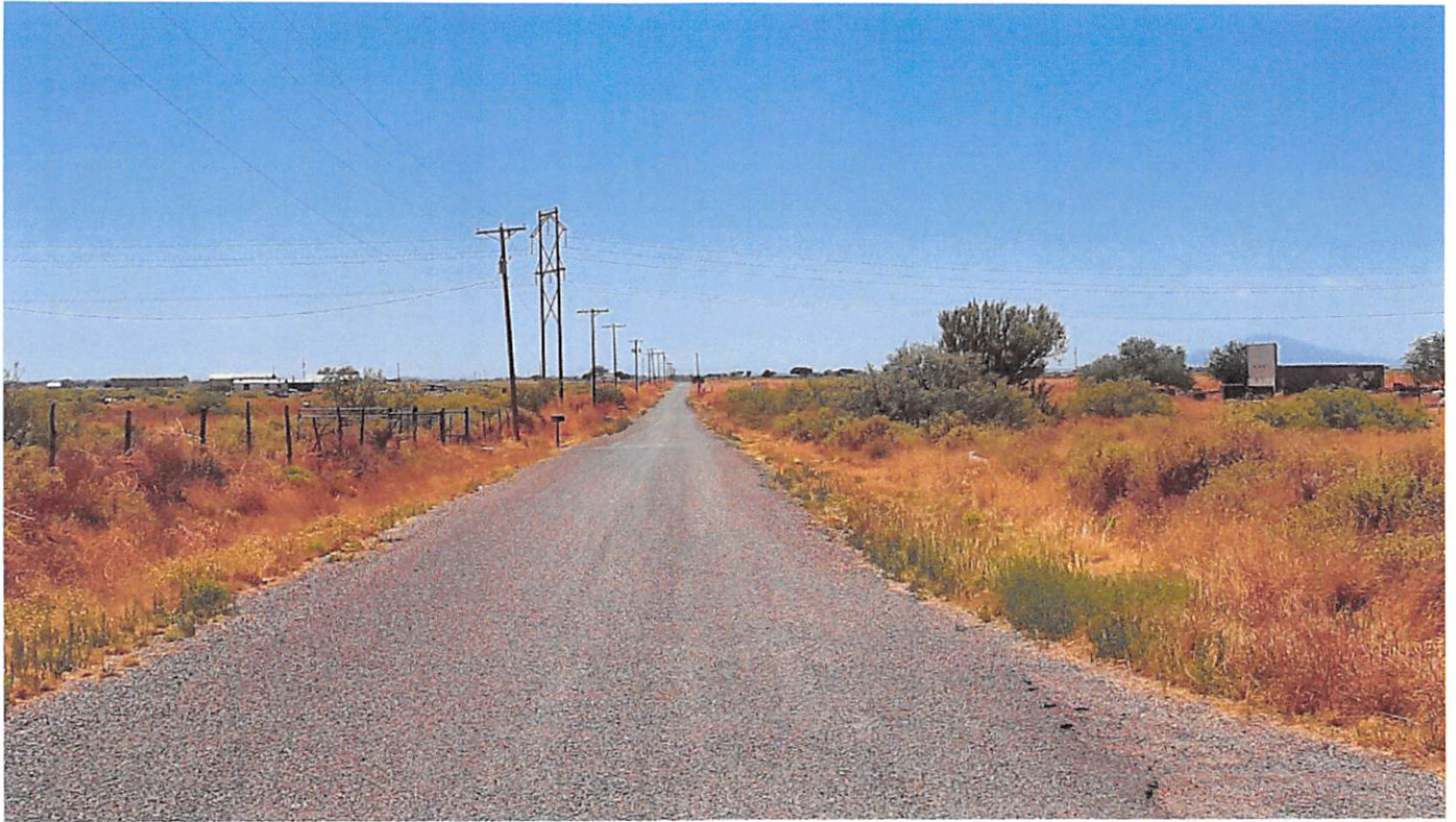
Zinnia Road looking east toward Red Bridge Road.
