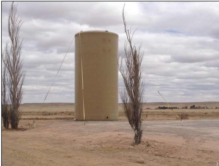
Figure 4.27. New 40,000 gallon water tank at the future site of Sierra Firestation 4, within the Tierra Grande subdivision.
