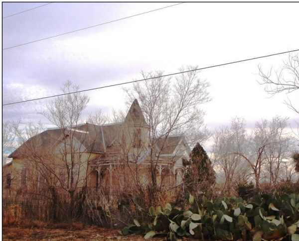
Figure 4.12. Derelict property with overgrown grounds.
