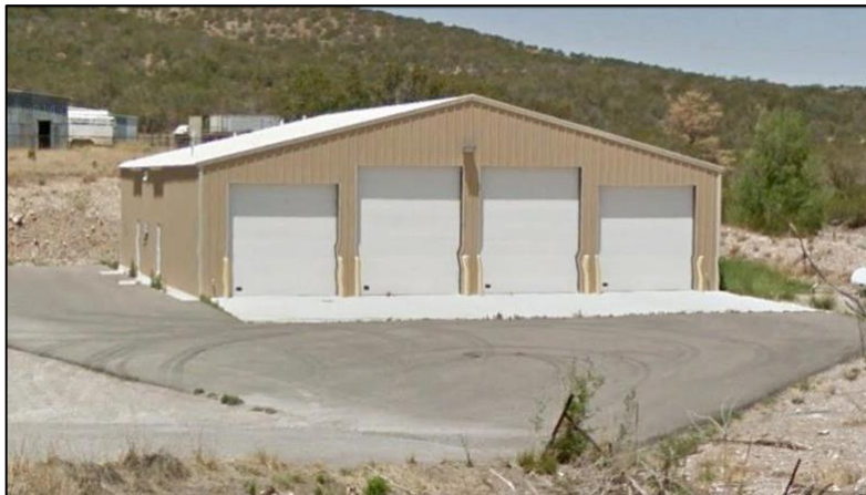
Figure 4.4. The new Peñasco Fire Station # 2.
