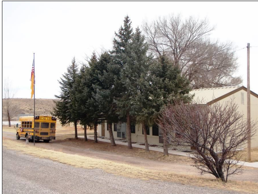
Figure 4.9. Elementary school at Dunken.
