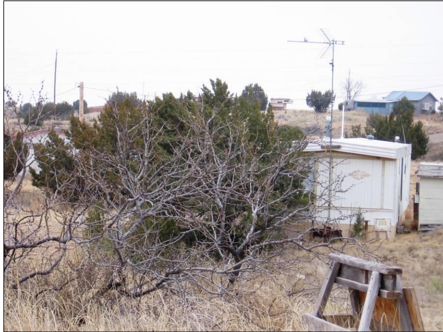
Figure 5.2. Structure requiring defensible space and fuels mitigation.
